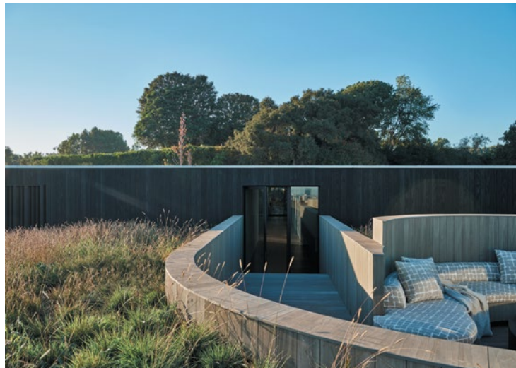
The shou sugi ban-clad residential level hovers above the battered stone wellness level created from Lichen limestone rubble.
